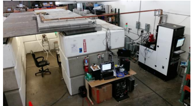
Figure 5: RadiaBeam radiation bunker. CPI klystron and magnetron modulator are on the right-hand side.
